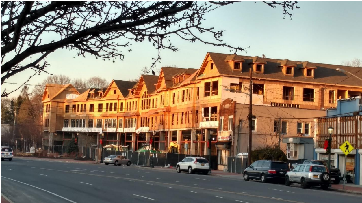
Gateway Plaza under construction
