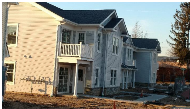
Columbia Terrace under construction
